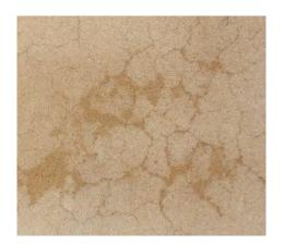
Crazing has been a concern since concrete has been in existence. The appearance of small cracks on the surface, especially when filled with water or dirt, can be alarming since it is assumed that the fissures are running through the entire cross section the concrete. But in general, crazing does not affect the structural integrity of the concrete and should not by itself be cause for rejection. All cement based products and many natural stones are susceptible to crazing.
